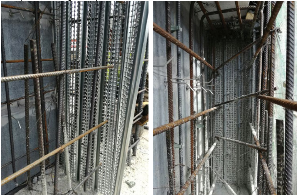
Example of a casting interruption in a wall.
