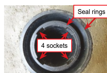
2 seal rings at the end of the cone + 4 sockets for grout retention using the Barnowitz method
