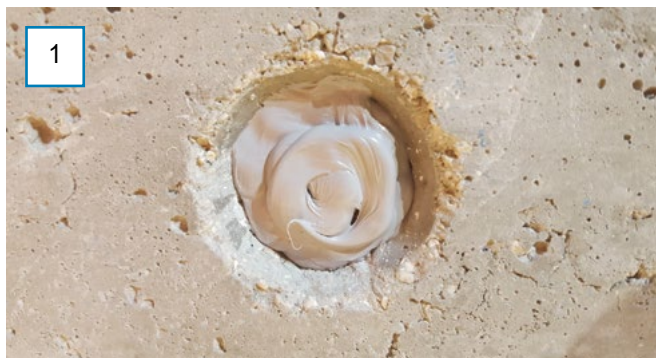
Injection of MS polymer glue into the Meriron pipe
