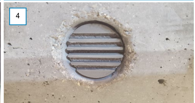
Stopper inside the concrete cone
