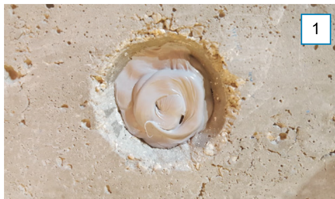
Inject polymer M5 glue into the Tie hole
